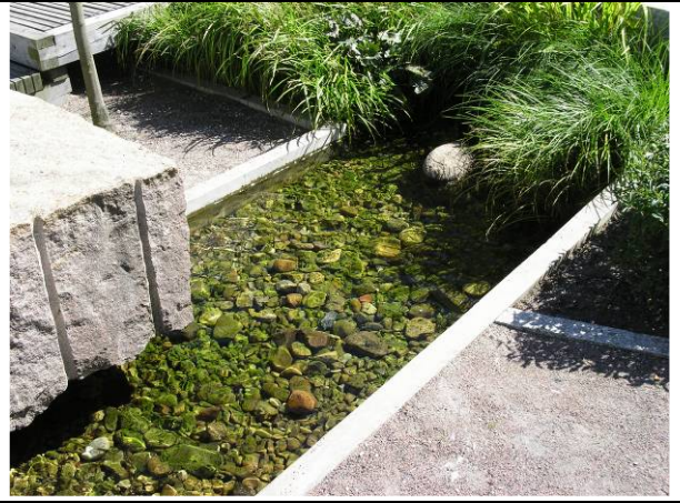
Watreco aeration system installed in Western Harbour (Malmo) since summer of 2005
